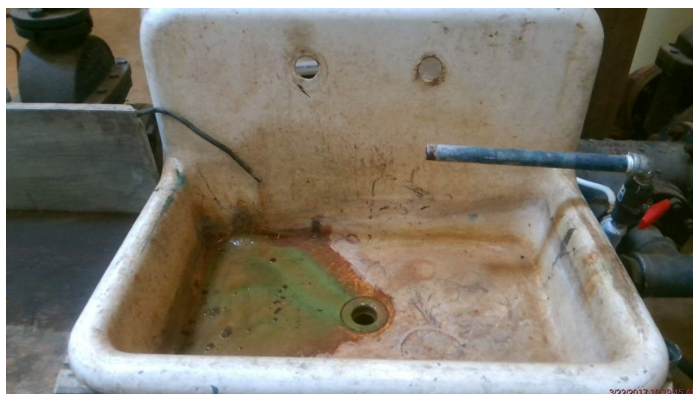
Copper pipe discharge from the clay valve vacuum relief without air gap
