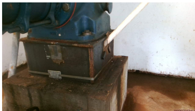
Openings in well casing with sounding pipe and unsecured screens
