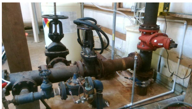
Well #1 chlorine injection and solution tank
