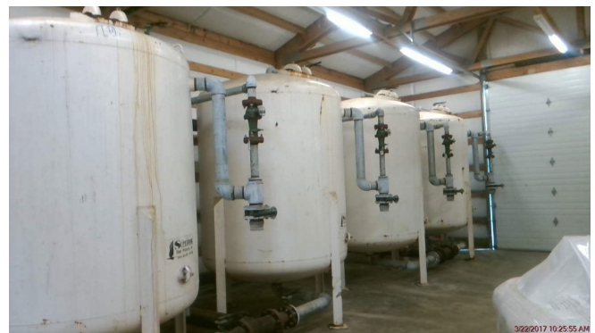
Well #3 calcite contactors
