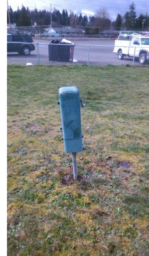
Locked and broken S04 sample tap
