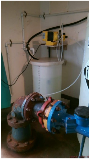
Well #3 chlorination injection
