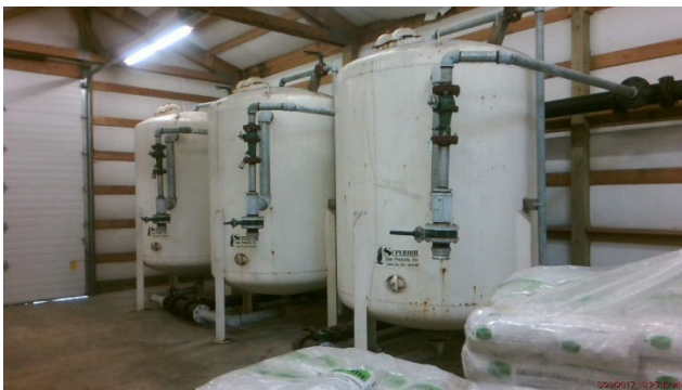
Well #1 calcite contactors
